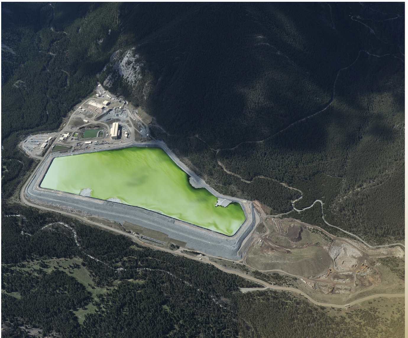
East Boulder Mine drainage
