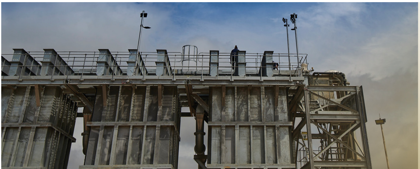
Water treatment plant located at the SA gold operations' Cooke 1 shaft area
