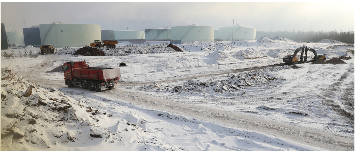
Keliber – starting earthworks for the lithium refinery in Kokkola, Finland
